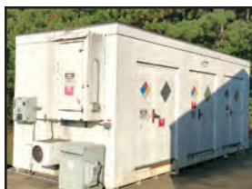
GFS HAZARDOUS LIQUID STORAGE UNIT
