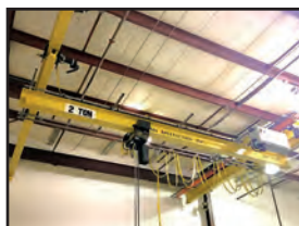
SPECIALTY SYSTEMS 2-TON BRIDGE CRANE
